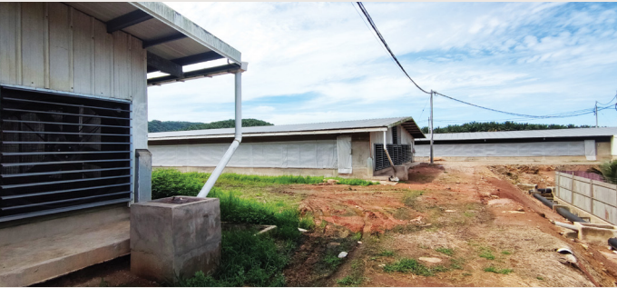
Rainwater harvesting system in QL Breeder
