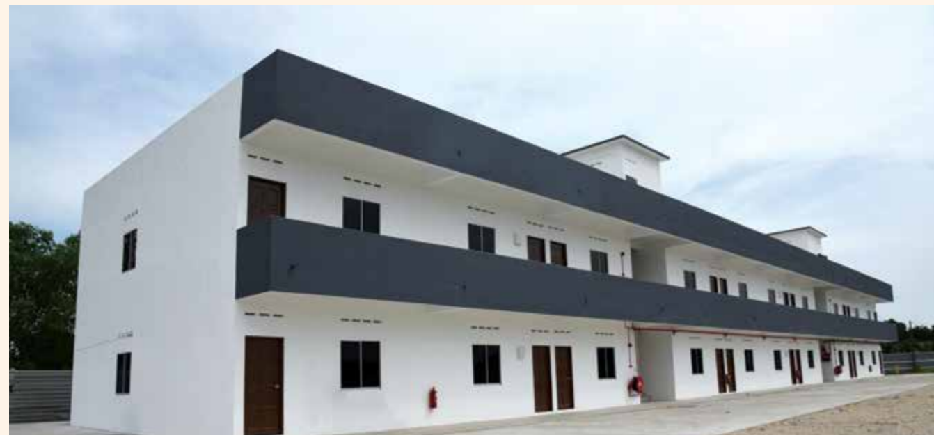
Newly-built workers' hostel in Endau, Johor.
