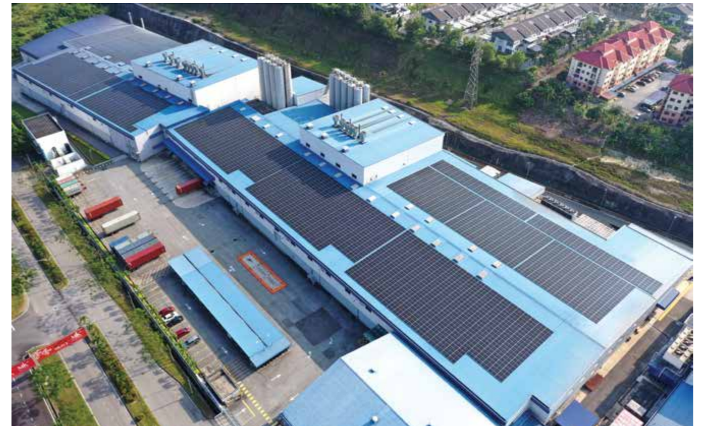
Rooftop solar panel installation at a customer's factory.
