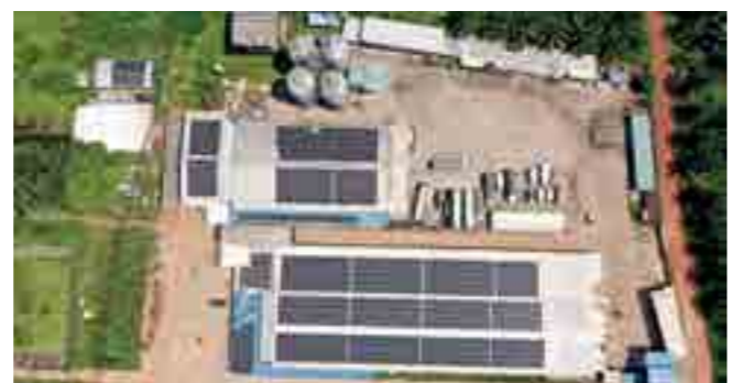
Solar Panels at QL Ansan Poultry Farm Sdn. Bhd., Rawang
