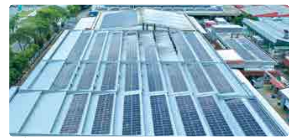
Photo of solar panels installation at QL Kitchen Sdn. Bhd.
